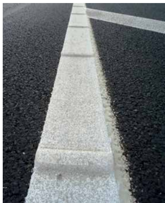
Form stable Profile Marking based on MMA
