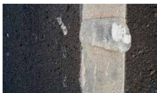
Profile marking based on thermoplastic road marking deformed within 1 year
